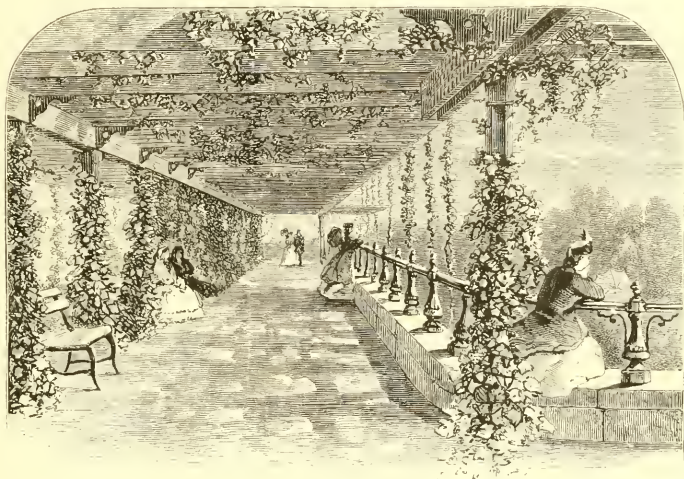
VINERY NEAR CASINO, OVERLOOKING THE MALL.
